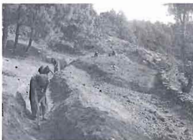
Drain work in Jwalamukhi Pond
