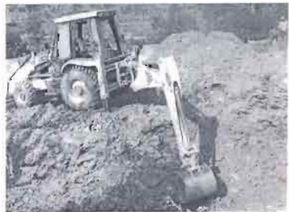
Excavation in Bhairabikot
