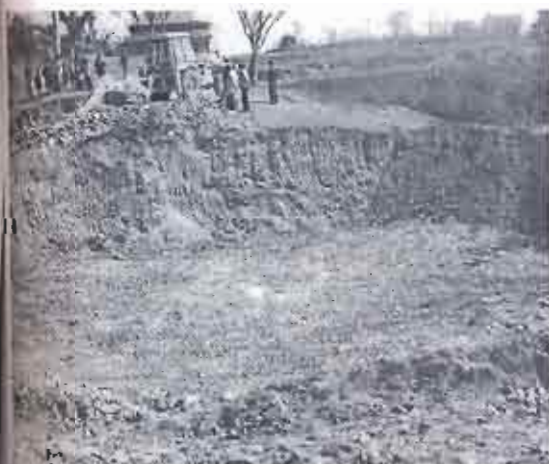
Excavation completion in Bhirabikot
