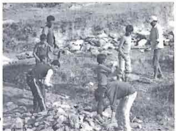
Stone collection for drain work
