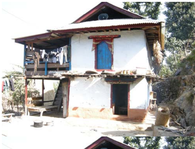
Figure 3 Beneficiary's house in Mukubung, Nagi-3, Panchthar
